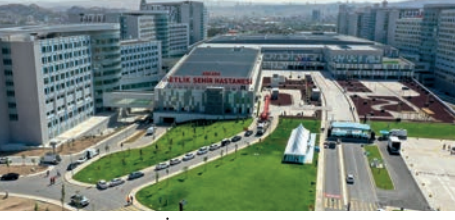
ETLİK CITY HOSPITAL
